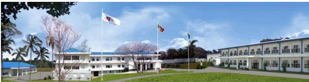
Figure 5.13 Flinth Industrial Park -Ranmuthugala Estate, Kadawatha
