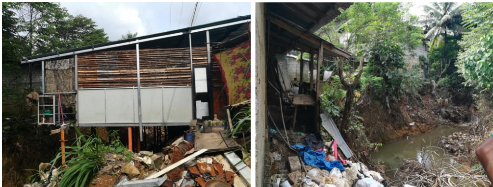
Figure 5.19 Sambawela Canal Reservations Encroachments
